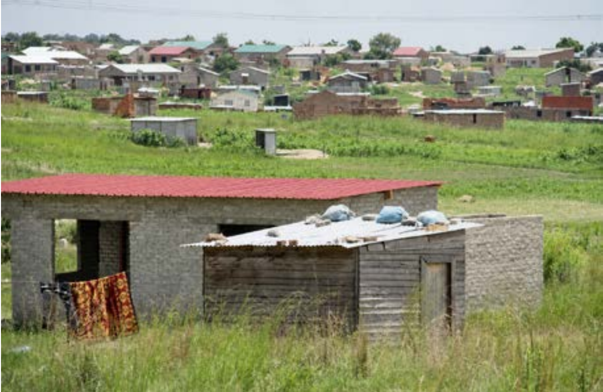
Unplanned houses occupying wetland areas in Epworth. The local authority says approximately 16,000 affected households could be relocated once its master plan is approved.
